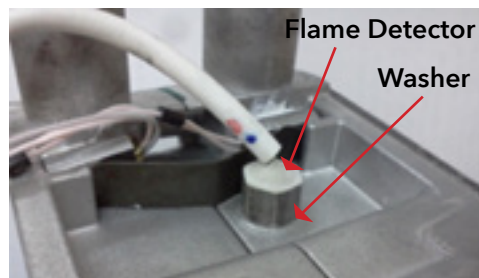
Fig. 6. Flame detector
